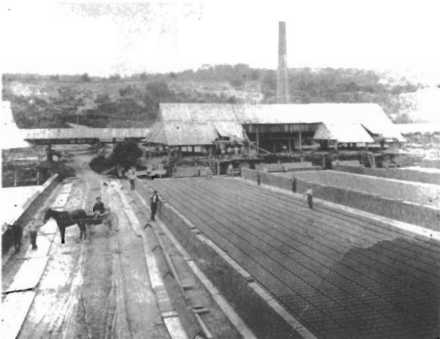
Hutton Co., c. 1900, showing drying yard, brick machine buildings and boiler flu. Courtesy Hutton Co.
