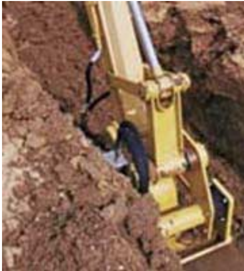
Vibratory Plate Compactor
